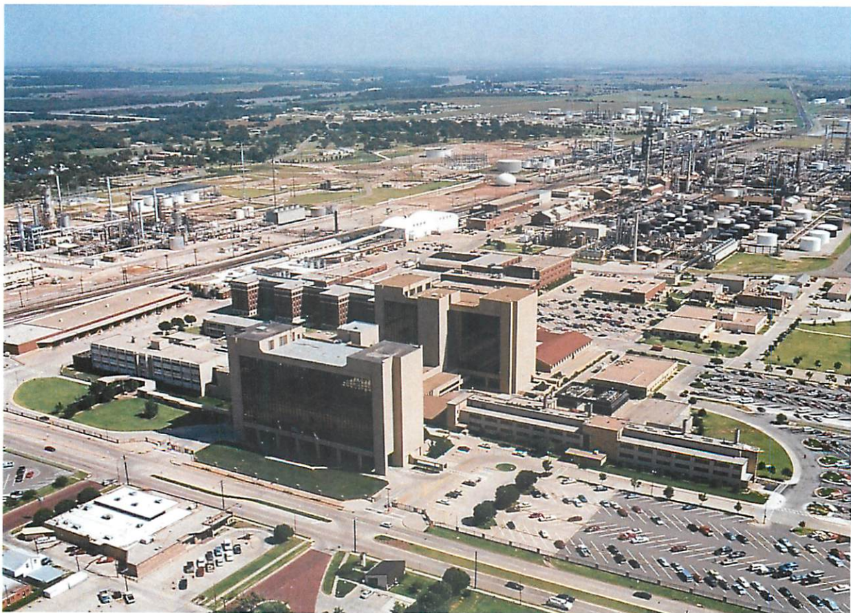
Pictured above, Phillips 66 employs an estimated 662 employees in Ponca City. The red brick building, southeast of the South Tower, is the original Marland Building, as it is still referred to today.
